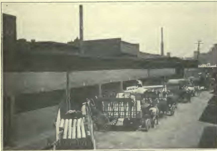
FIG. 314. FREIGHT HOUSES. Loading Platform of the Freight House of the Michigan Central Railroad, at the South Water Street Yard, Chicago.
